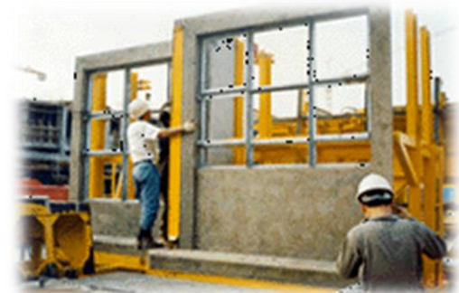
Precast concrete facade
