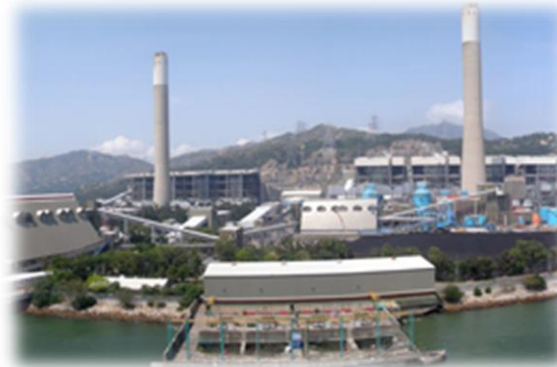
CLP – Castle Peak Power Station
