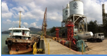
Heavy Loading Berth - Load ash to barge
