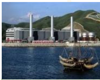
3 * 100MW Penny's Bay Power Station IDO
