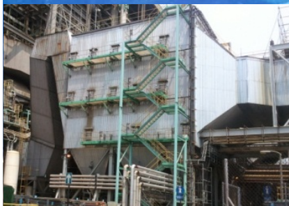
Electrostatic Precipitators (ESP) - Collect PFA from flue gas
