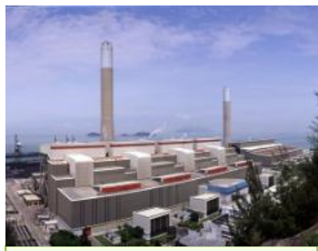
4 * 677MW, 4 * 350MW Castle Peak Power Station Coal Fired
