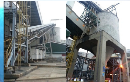
ACC & FBA silos - Collect & store FBA - Truck loading facilities
