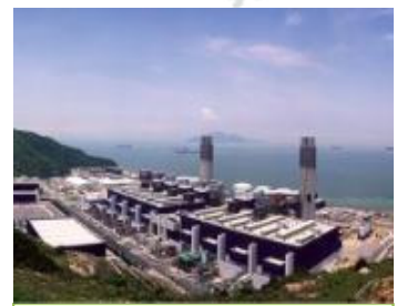
8 * 312.5MW Black Point Power Station Natural Gas
