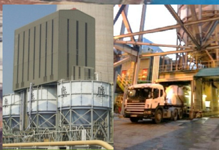
Ash Classification Plant (ACP) - Separate fine PFA from coarse PFA - Storage for both Classified PFA and Reject - Ash Tankers loading facilities
