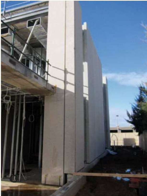
Library built with AAM precast walls
