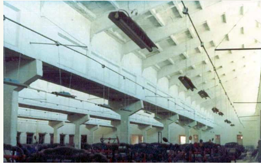
Beam & Columns of workshop
