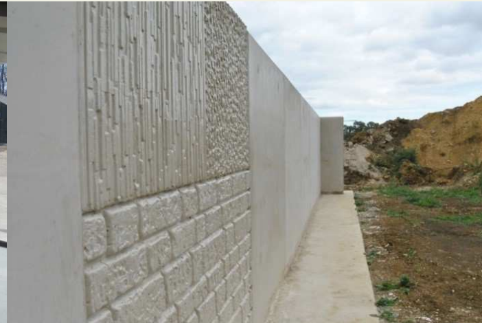
Insitu Wall (No Joint) 34m Long
