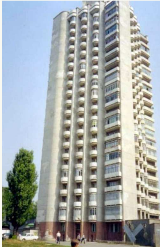
24-storey building from insitu and precast AAM concrete
