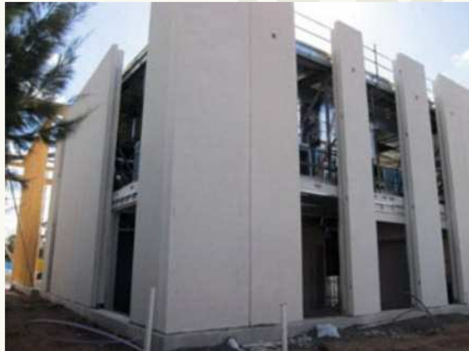
Library built with AAM precast walls
