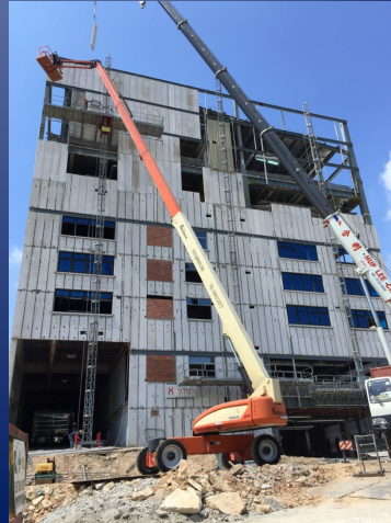
Industrial building @ Sungei Kadut
